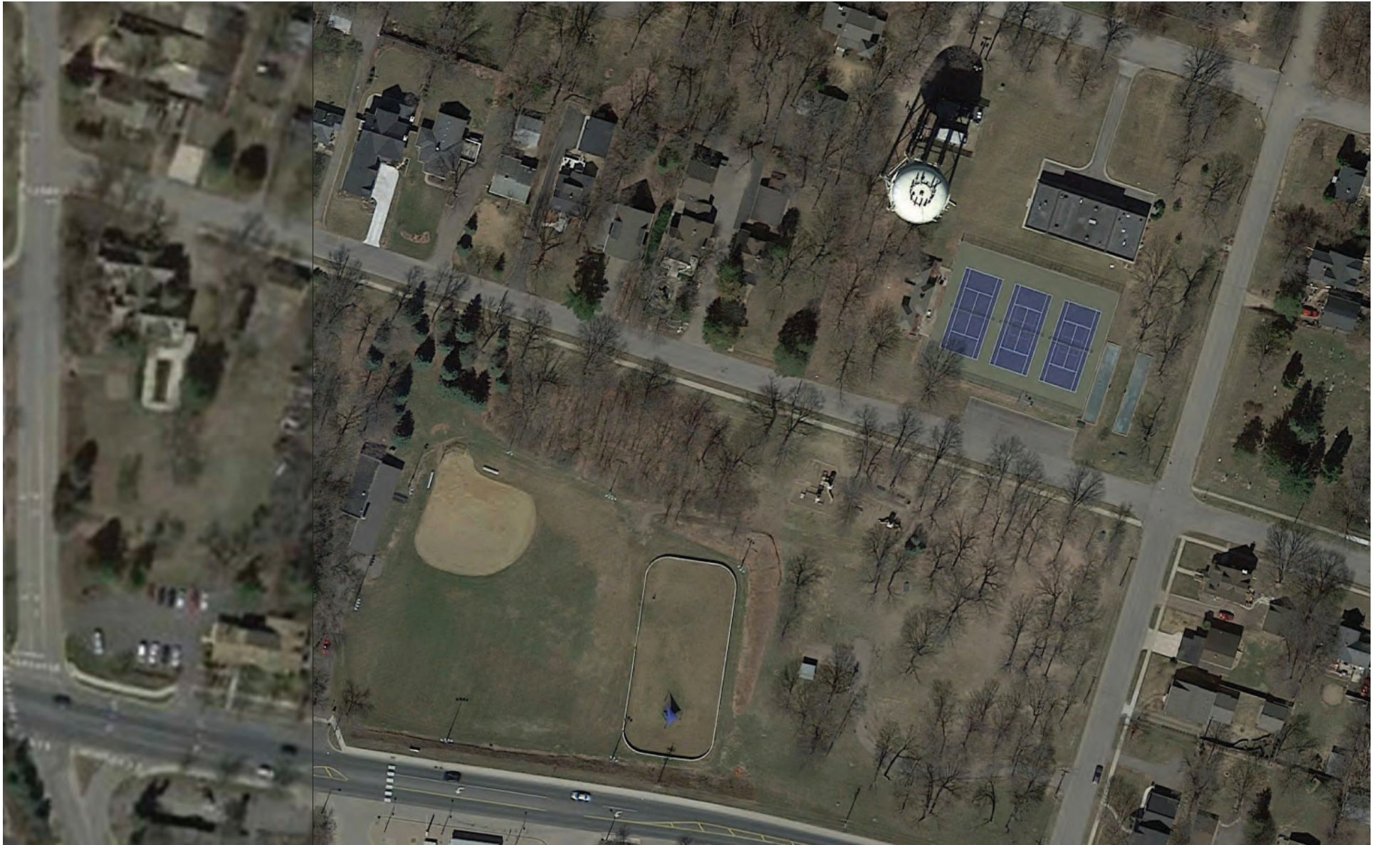
KLAPPRICH PARK + BELL COURTS EXISTING CONDITIONS
