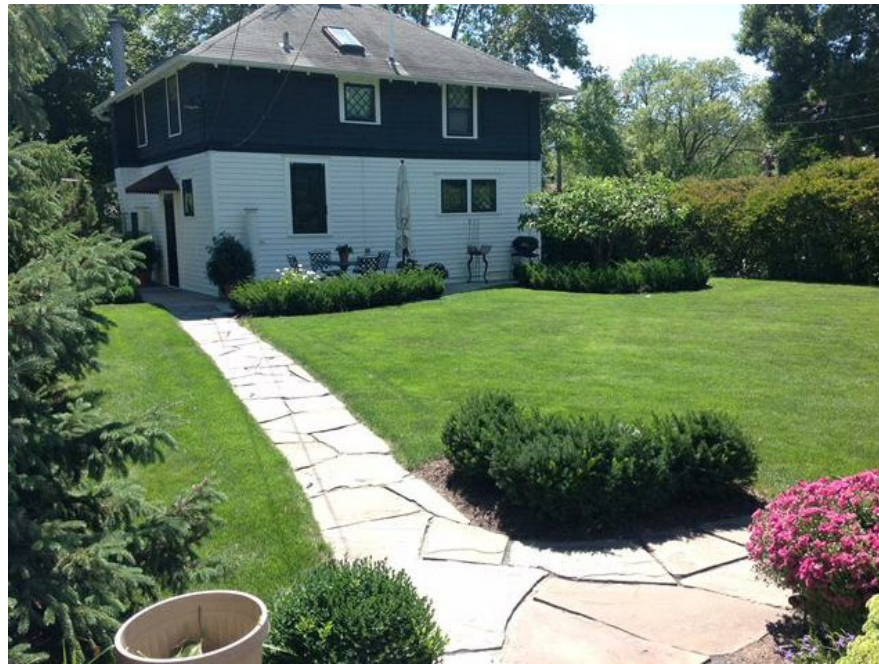
EXISTING NORTH FACADE
