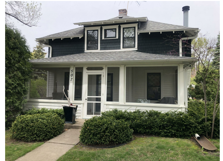
EXISTING SOUTH FACADE
